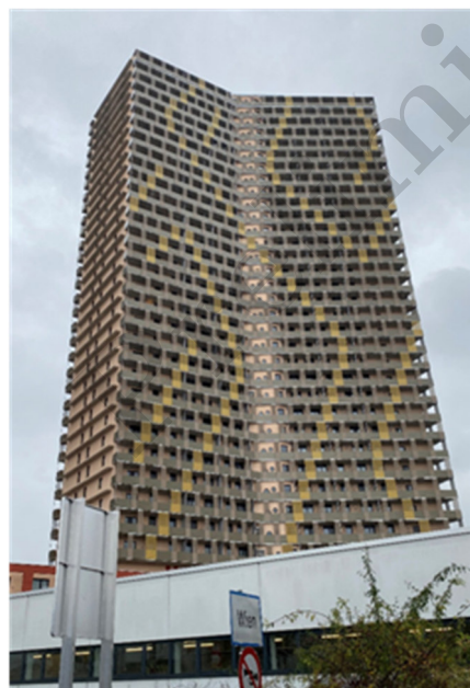
Figure 7. Example of a high-rise building with balconies
