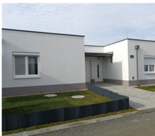
Figure 6. Example of a bungalow, small façade with a recess
