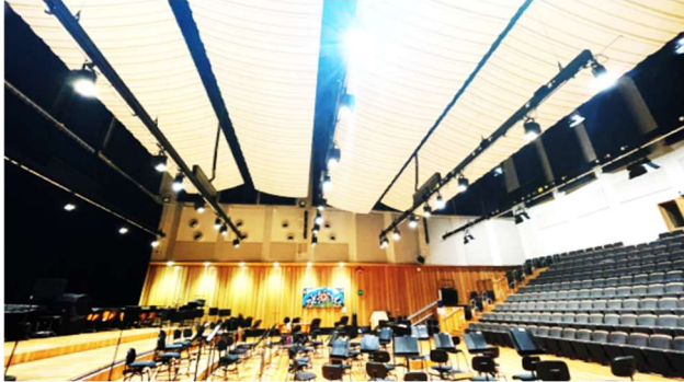
Figure 1. Photo of the studio showing the large reflectors above the orchestra and deployed absorption above the audience seating.
